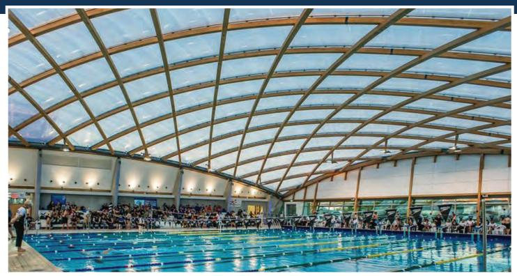
Texlon<sup>®</sup> ETFE is one of the most sustainable high performance cladding technologies in the world. The efficiency and lightness of the Texlon system uses less embodied energy, is exceptionally durable, recyclable, and energy efficient; helping reduce the buildings overall carbon footprint.
