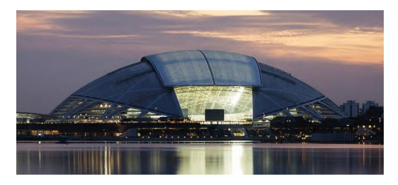
The Texlon® system's multi-layered construction allows us to incorporate graphics, add color, and even incorporate LED lights. These "intelligent" roofing systems are engineered to span great distances of any size and can be designed to any shape that fits your needs, providing an infinite number of possibilities to design buildings of iconic visual presence.
